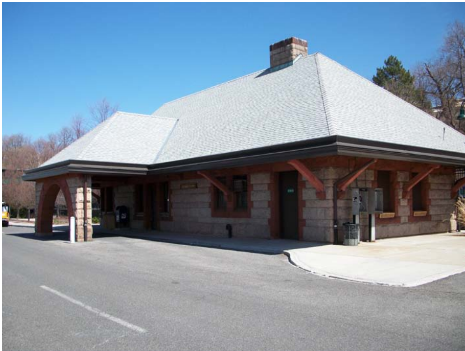
West Side of Building
