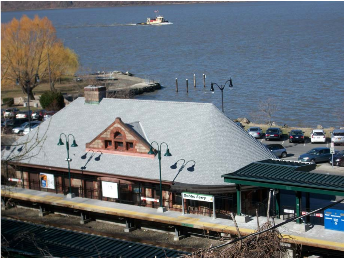
East Side View of Building
