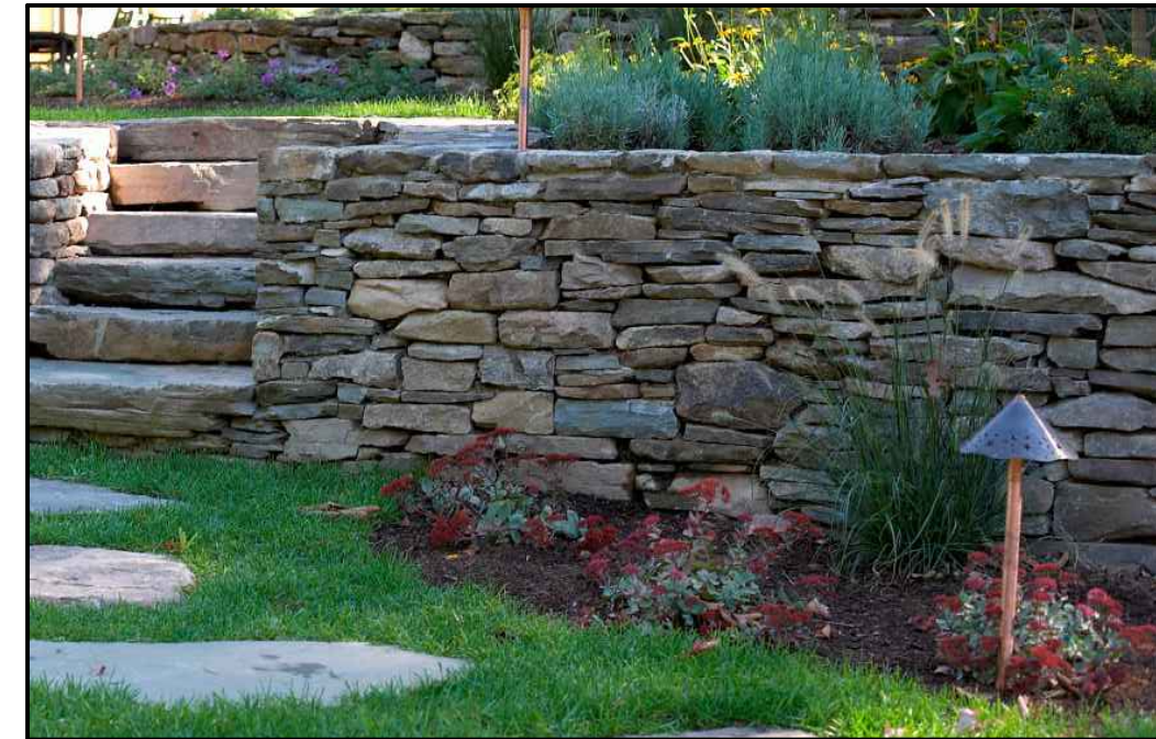
E-ST-1 NEW DRY STACK STONE ON WALL
