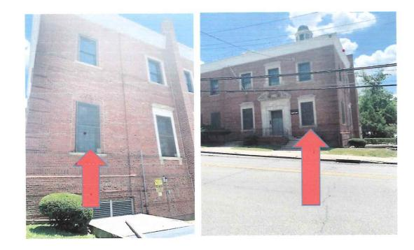
Existing window to be removed & replaced with new louver. The same screen on the exterior window as shown in picture above will be installed on the exterior of new louvers. There is no change in window size 48"W x 96"H. Color of new louvers to match existing picture as shown below. New louver size 48"Wx96"H. Please see attached approved past submittal from Pottorf manufacturer.
