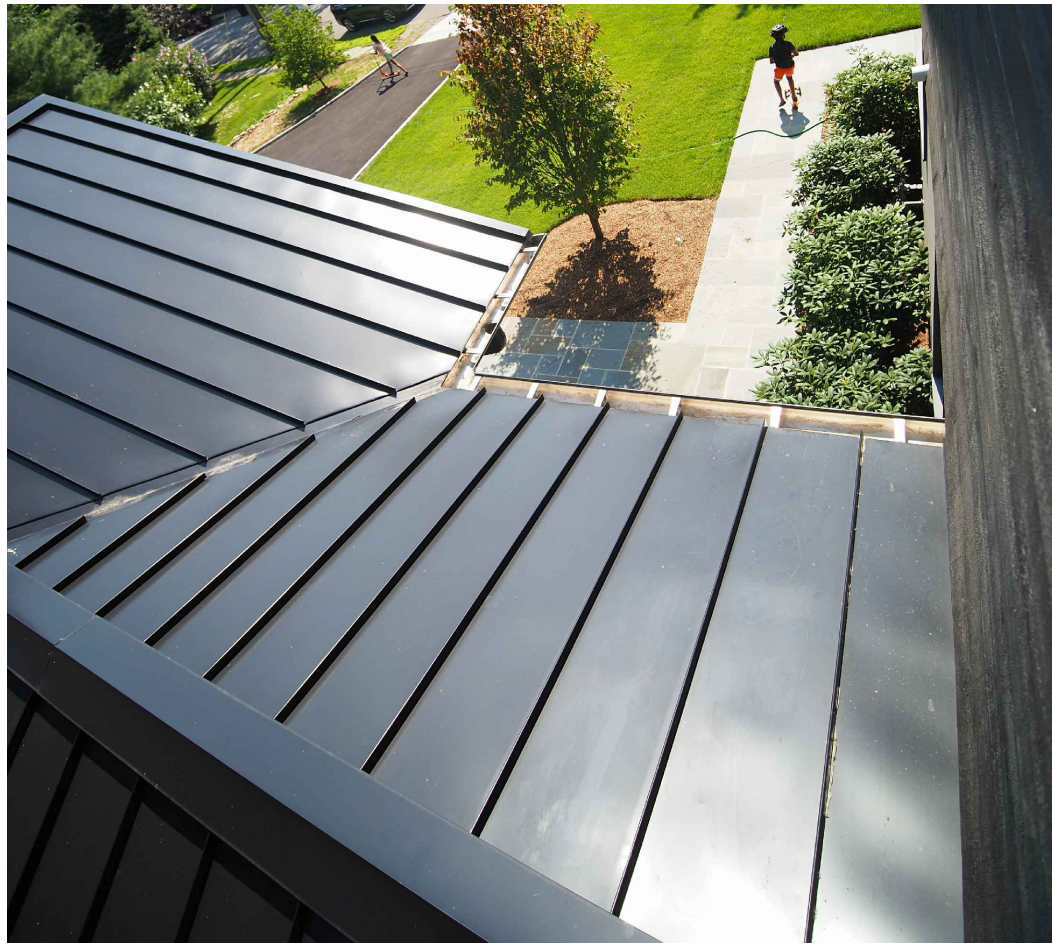
PAC-CLAD STANDING SEAM METAL ROOFING (GRAPHITE FINISH PROPOSED, MATTE BLACK SHOWN)
