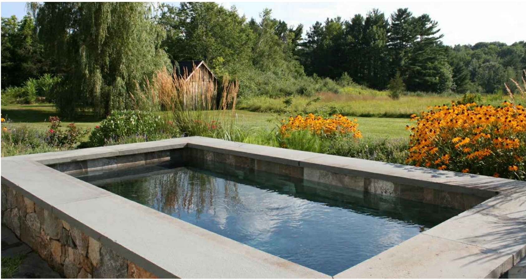
RAISED SOAK POOL WITH STONE SURROUND, THERMAL BLUESTONE COPING
