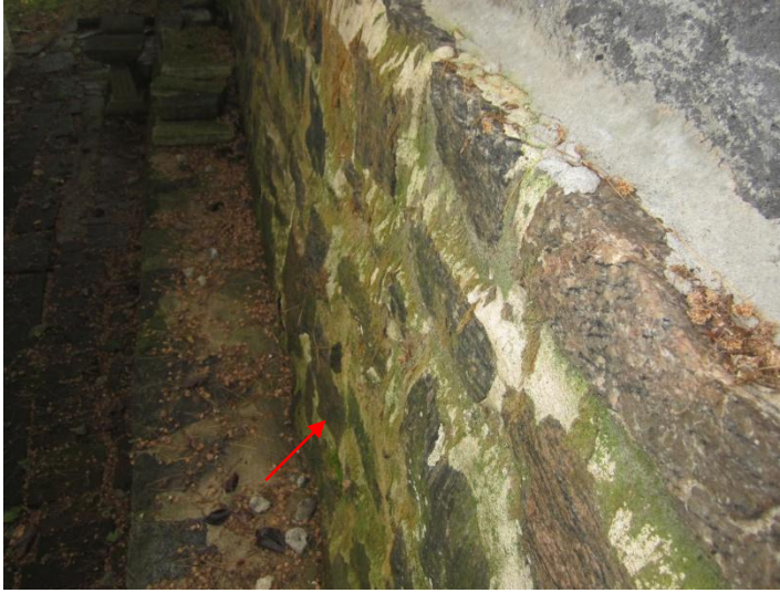
Stone wall at base was found to be sound and free of major deformation.
