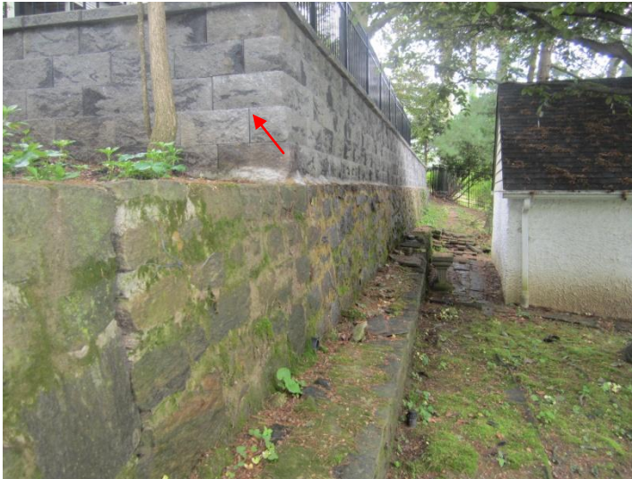
Walls are independent, and has proper return.
