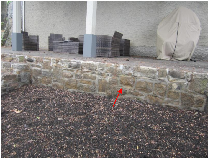
Patio retaining wall is sound.
