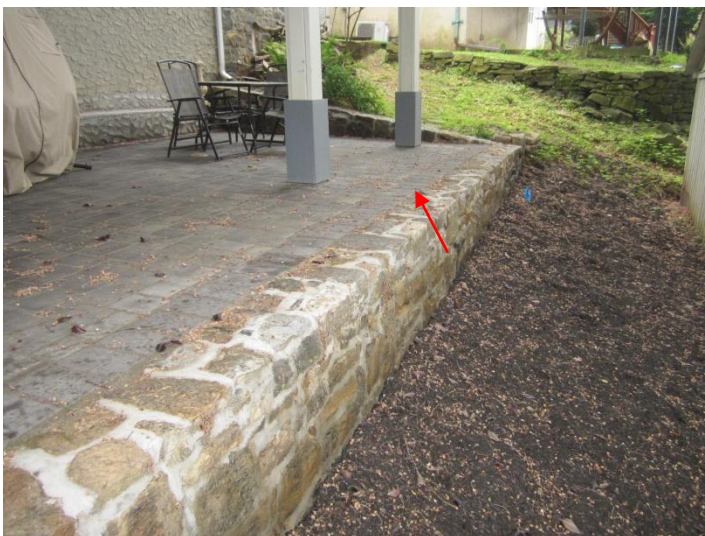
A safety railing of should be installed around the perimeter of the patio. The railing should measure at least 36" inches above the patio floor level.
