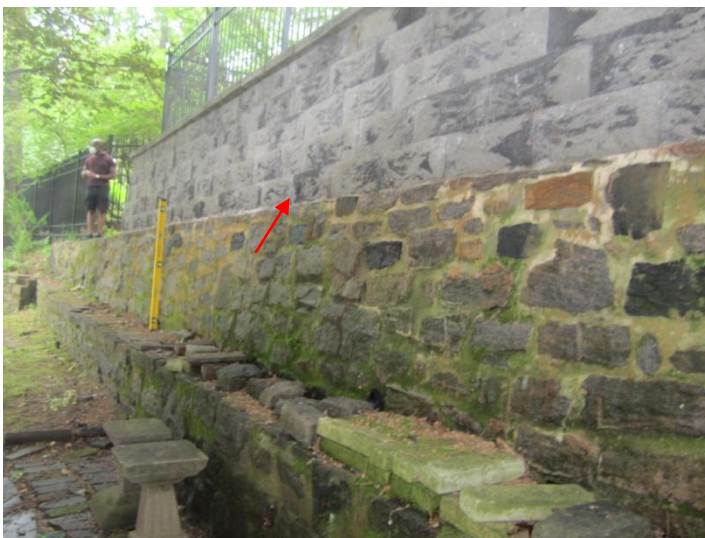
Walls are constructed independant of each other.
