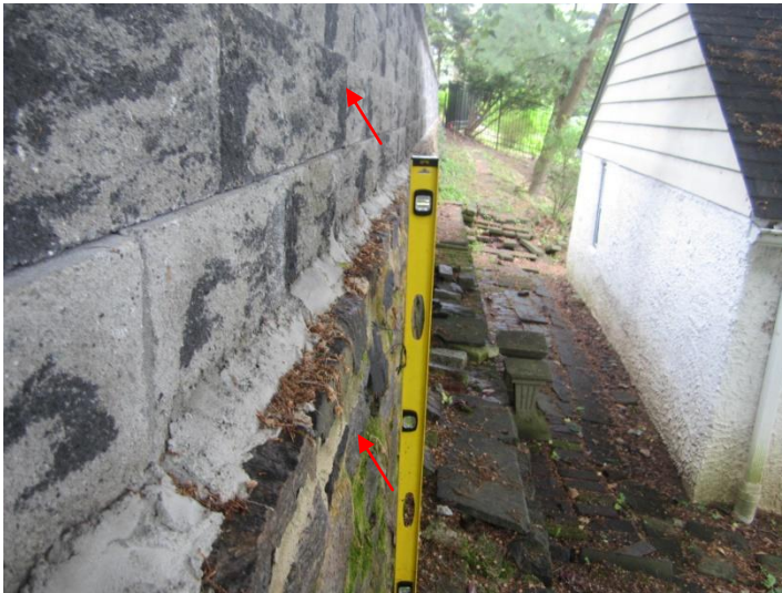
View of retaining wall looking to the South. Both upper new wall and lower original wall are properly installed with proper inward batter angle.
