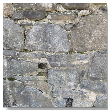
PALISADE ST RETAINING WALL FIELDSTONE
