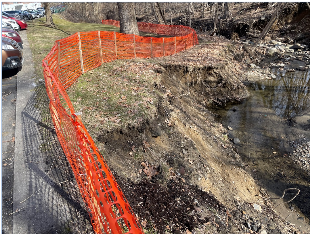
Photograph 4 – Eroded Western Bank of Wicker's Creek Adjacent to Condominium Complex Parking Lot, Looking North. (Image Dated 03-15-2022)
