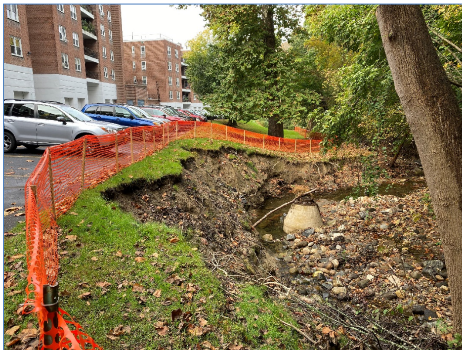
Photograph 1 – Eroded Western Bank of Wicker's Creek Adjacent to Condominium Complex Parking Lot, Looking North. (Image Dated 10-25-2021)
