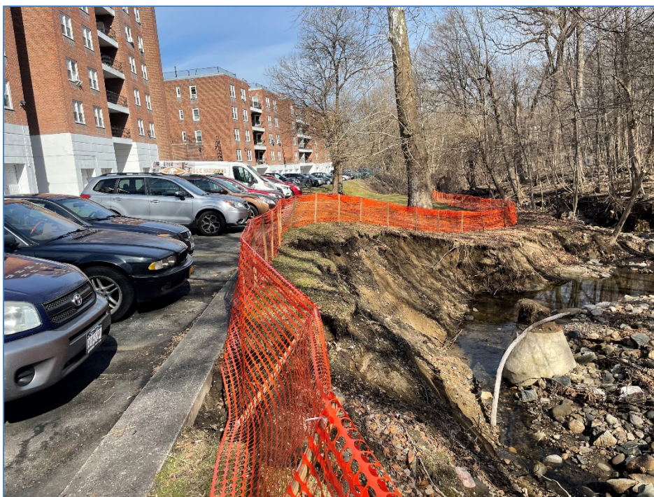
Photograph 2 – Eroded Western Bank of Wicker's Creek Adjacent to Condominium Complex Parking Lot, Looking North. (Image Dated 03-15-2022)
