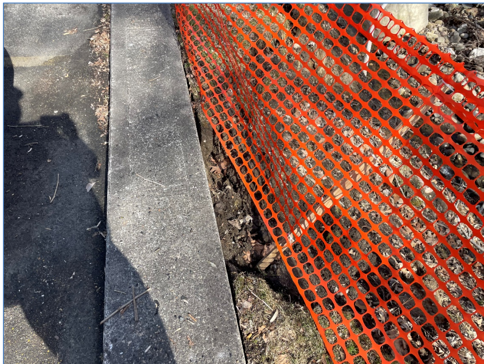
Photograph 3 – Eroded Western Bank of Wicker's Creek Abutting Concrete Curb, Looking North. (Image Dated 03-15-2022)
