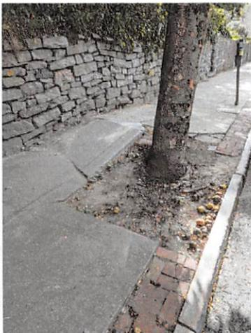
PHOTO 5: BARE SOIL AND SIDEWALK HEAVE AT EXISTING TREE PITS
