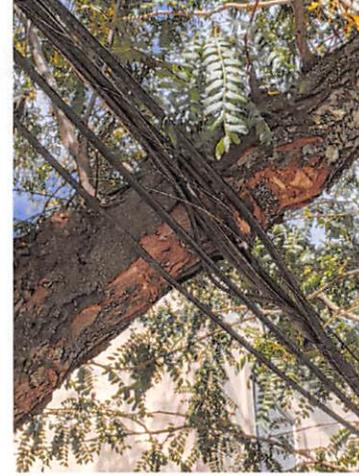
PHOTO 3: OVERHEAD WIRES IMPACTING TREE LIMBS
