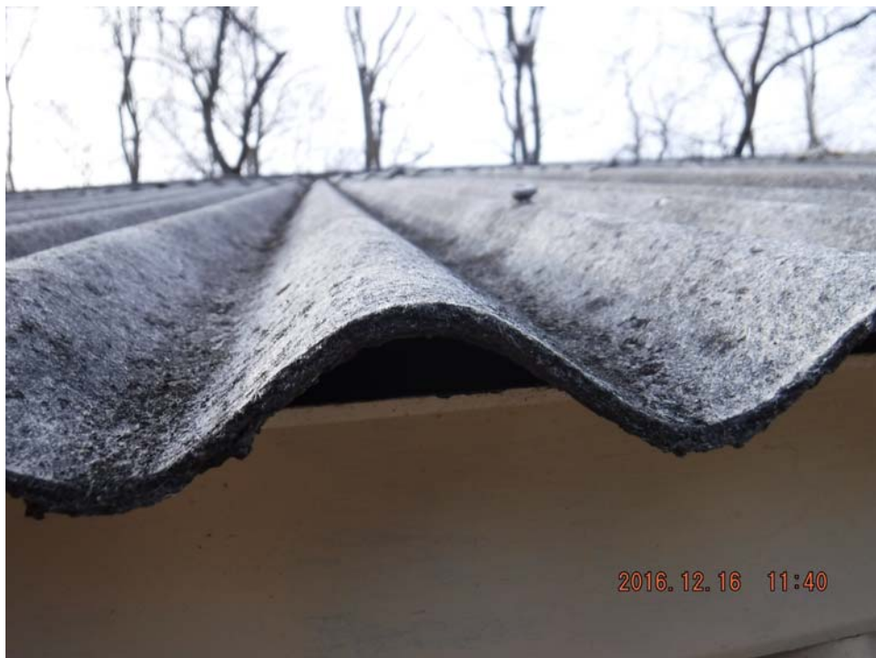
Roof, asbestos containing roof transite.
