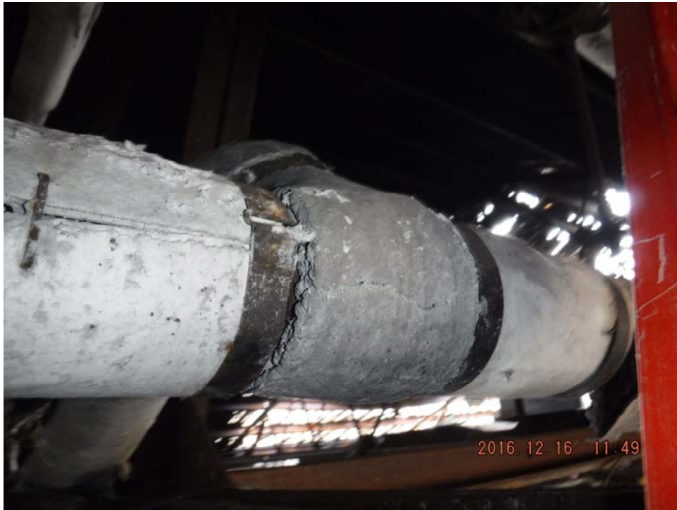
Interior, asbestos containing pipe fitting and insulation
