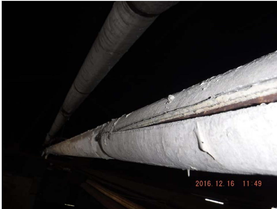
Interior, asbestos containing pipe insulation.
