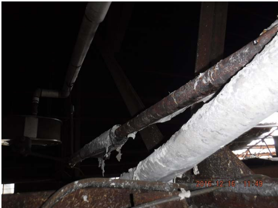
Interior, asbestos containing pipe insulation.
