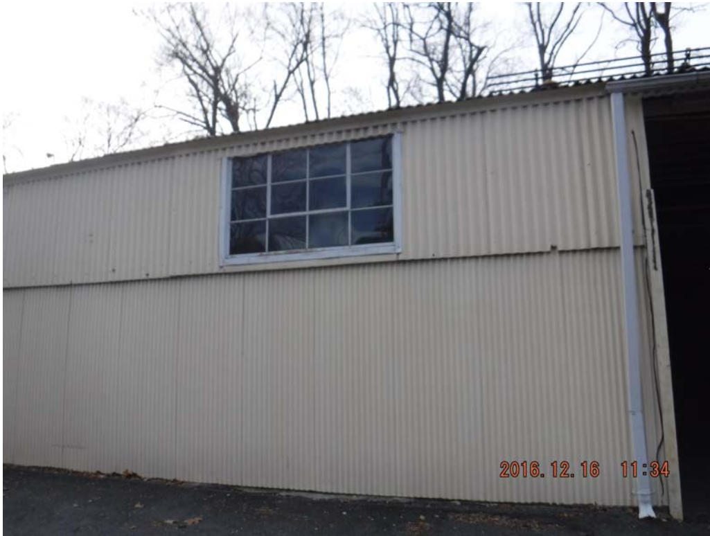
Siding, asbestos containing transite siding
