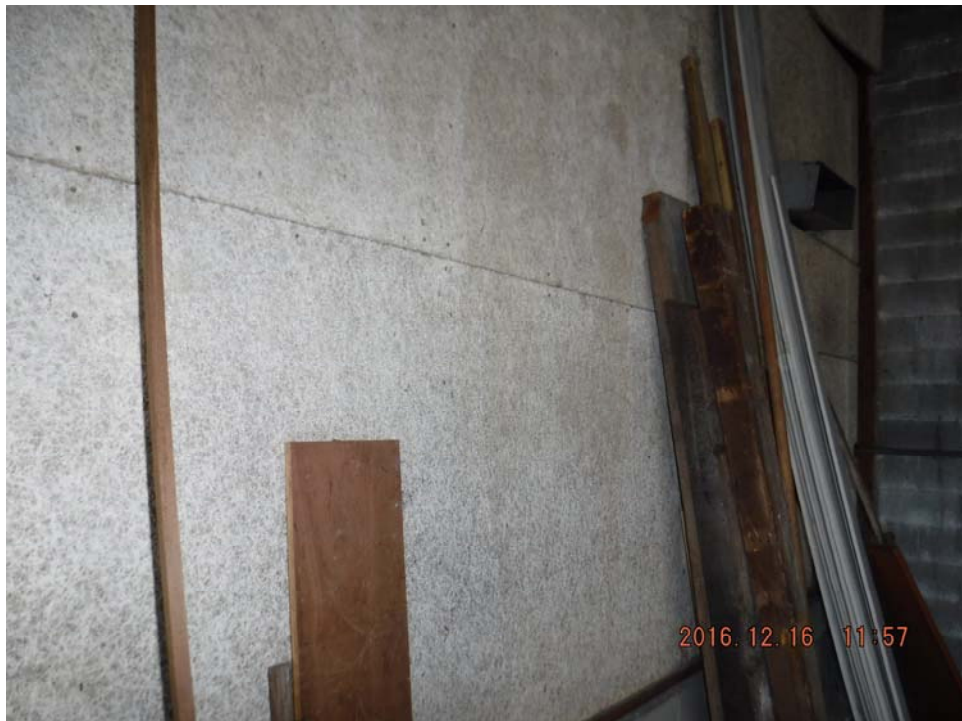
Interior, non-asbestos containing wall finishing material.
