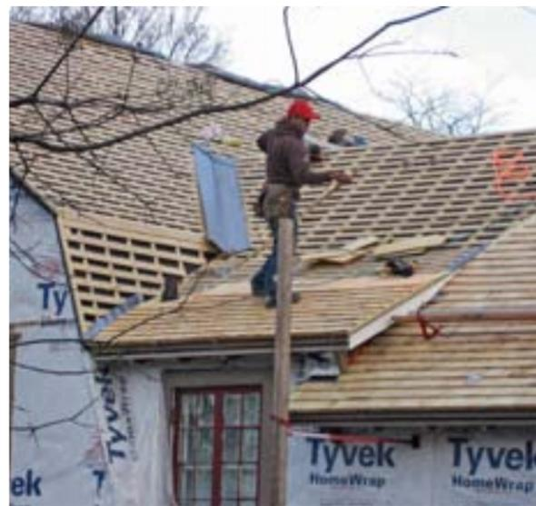
Traditional roof furring or equivalent spacer systems provide ventilation for the shingles above. Ventilation under cladding to promote drying enhances the longevity of insulated walls and roofs, which used to be dried by waste heat through uninsulated walls.
