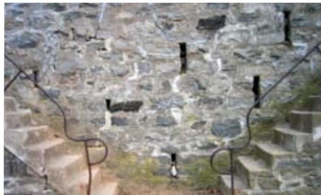
*Age-old retaining wall and steps. Random weep holes deal with underground water pressure.*
