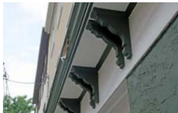
Brackets provide a graceful transition at eaves and overhangs. Wood details are traditional; plastics and composites can lead to problems due to their greater expansion and contraction properties.
