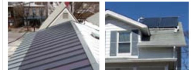
Thin-film solar collectors laminated onto a metal roof (left) are much better suited than high profile arrays facing the street in a historic district.
