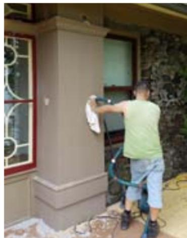
Dense-pack cellulose, here being pumped in from the exterior, is a relatively low cost recycled product suitable for retrofit of old and historic buildings. It has a lower climate change impact than foam insulations.
