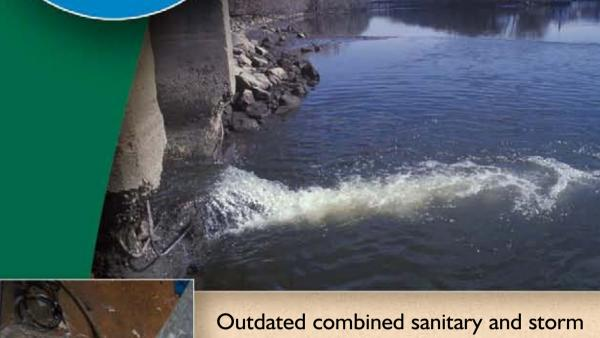
Outdated combined sanitary and storm sewer systems can overflow, causing combined sewer overflows (CSOs).
