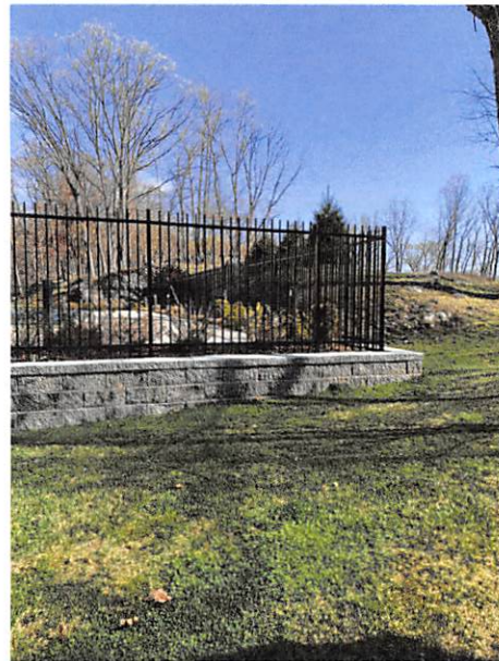
5 - EXISTING RETAINING WALL AT POOL AREA
