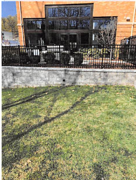
5 - EXISTING RETAINING WALL WITH DRAIN AT BBQ AREA
