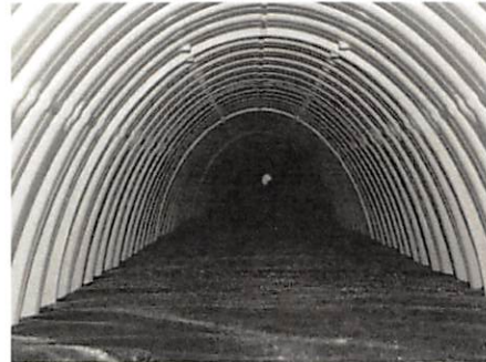
Looking down the Isolator Row
