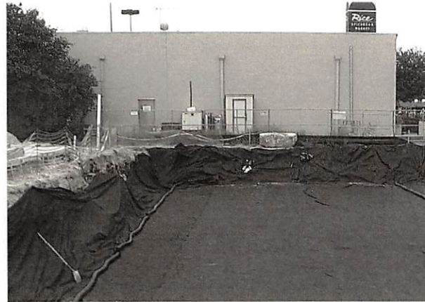
Place non-woven geotextile over prepared soils and up excavation walls.
