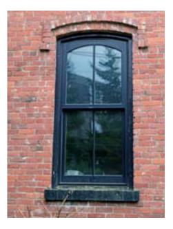
The arch-top effect was often achieved with less effort within a square upper sash behind curved trim, as in this case. The brick window hood above both helps shed water and enhance the appearance. • When installing new or replacement windows, install true or simulated divided-light muntins rather than snap-in or flat muntin grids.
