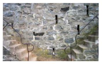
Age-old retaining wall and steps. Random weep holes deal with underground water pressure.
