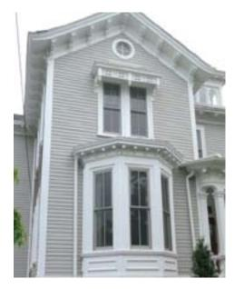
Exterior details work together to reinforce the basic volumes and create the style of the building, In general, decoration, as in brackets. window hood and moldings shown here, is applied to horizontal elements at a scale appropriate to each.
