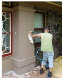
Dense-pack cellulose, here being pumped in from the exterior, is a relatively low cost recycled product suitable for retrofit of old and historic buildings. It has a lower climate change impact than foam insulations. The most cost-effective green strategies such as insulation and air sealing do not dictate architectural style or prevent new buildings from fitting their context. Some knowledge is required to properly apply these techniques to existing buildings of any era.
