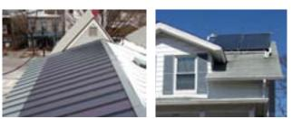
Thin-film solar collectors laminated onto a metal roof (left) are much better suited than high profile arrays facing the street in a historic district.
