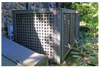
Air circulates through lattice enclosure hiding meter and air conditioning. Lattice is painted to blend with house palette.
