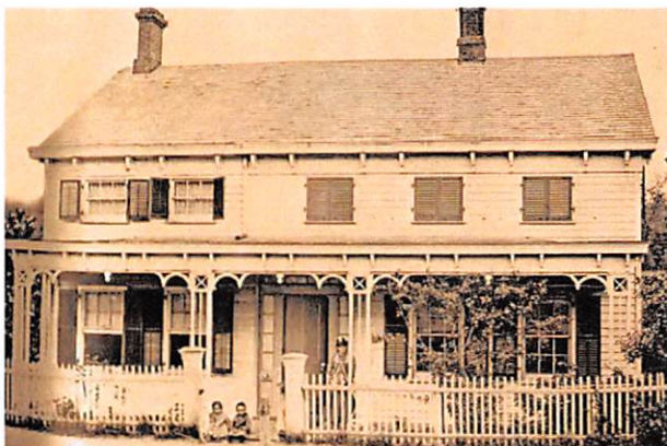
An earlier incarnation of 66 Cedar Street had 5 bays, two chimneys and an ornate later shallow porch.
