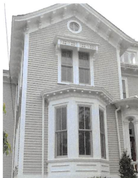
Exterior details work together to reinforce the basic volumes and create the style of the building. In general, decoration, as in brackets, window hood and moldings shown here, is applied to horizontal elements at a scale appropriate to each.
