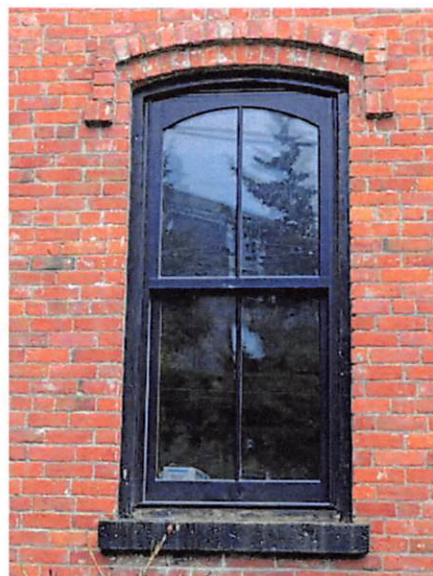
The arch-top effect was often achieved with less effort within a square upper sash behind curved trim, as in this case. The brick window hood above both helps shed water and enhance the appearance.
