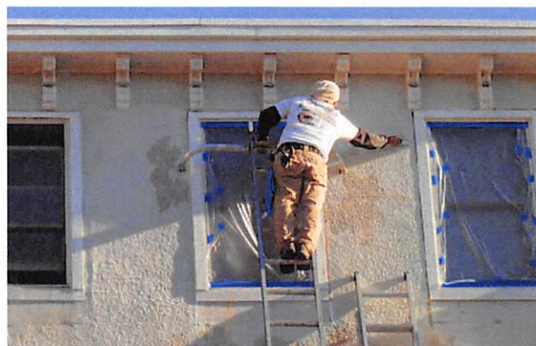
Integral color in stucco mixes makes patching more seamless when required.
