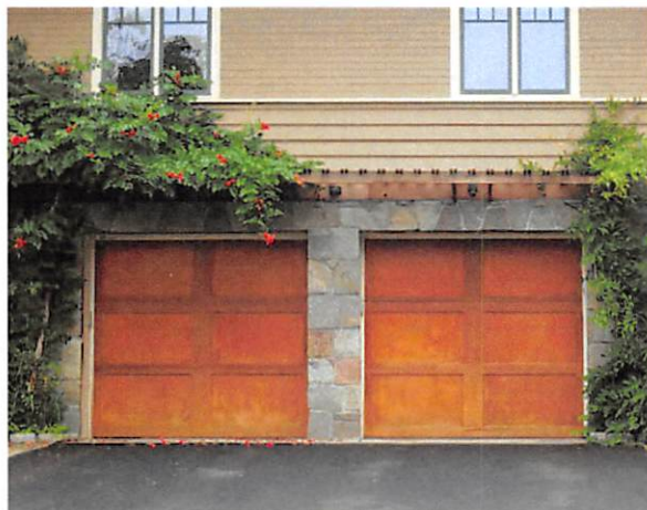
Prominent garage doors can detract considerably or, as above, be better integrated into a building's design through the choice of material, pattern, color and surrounding architectural treatments like trellises and vines shown here.
