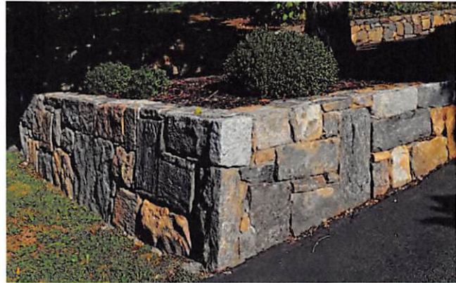
Dressed stone retaining wall; mortared joints.
