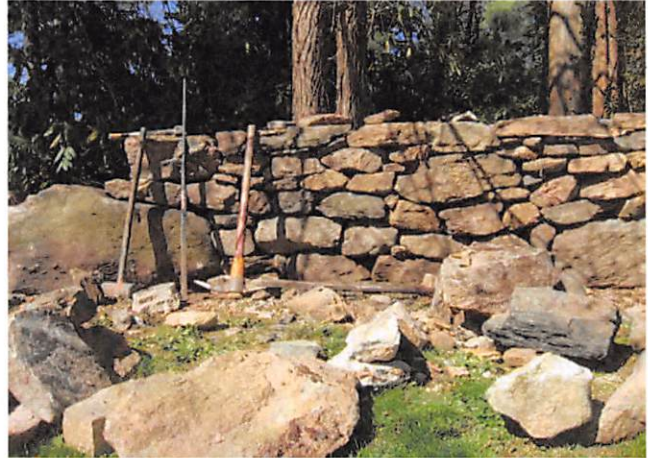
In construction: Rustic wall shaped around existing boulder.
