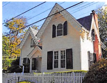
Tracery plays with light and shade and emphasizes the gables in this "Carpenter Gothic" cottage. Flat topped upper windows are a variant.
