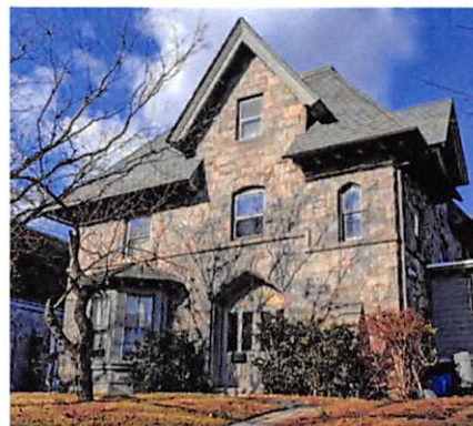
This example combines pointed arches on doors and windows with flat arches. Steep gables are enhanced by deeply sculpted trim.
