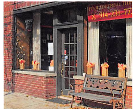
Traditional divided doors and trim fitting the building can co-exist with traditional plate glass storefront windows.
