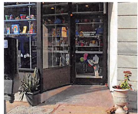
Ramped recessed entries are user-friendly. Clean modern storefronts can be inserted in historic buildings if original materials have disappeared.
