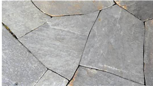
Terrace surface: stones shaped to minimize joint size.
