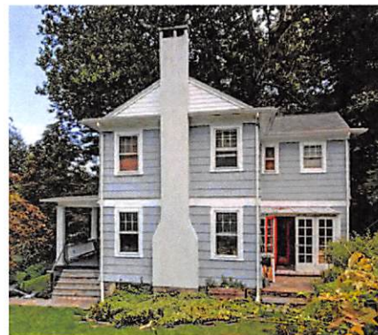
Overhangs with Craftsman and Prairie Style horizontal emphasis combine here with a traditional Colonial Revival approach.
