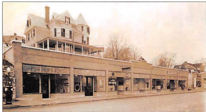
Downtown retail shops form a new street wall in front of older houses set back on the property: a classic American downtown sequence. (Robison house c. 1927)
