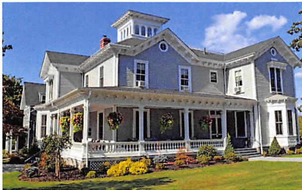
An arch-windowed belvedere provides a tower form at a corner of an upper flat roof. Heavy bracketed roof overhangs and elaborate window shrouds add decorative flourishes. A wrap-around porch shades southern and western exposures. Small circular windows punctuate the gables.
