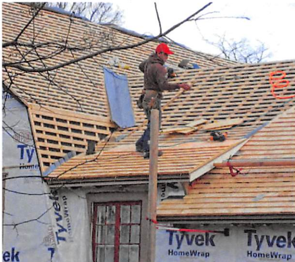
Traditional roof furring or equivalent spacer systems (e.g. “Ventgrid”) provide ventilation for the shingles above. Ventilation under cladding to promote drying enhances the longevity of insulated walls and roofs, which used to be dried by waste heat through uninsulated walls.
