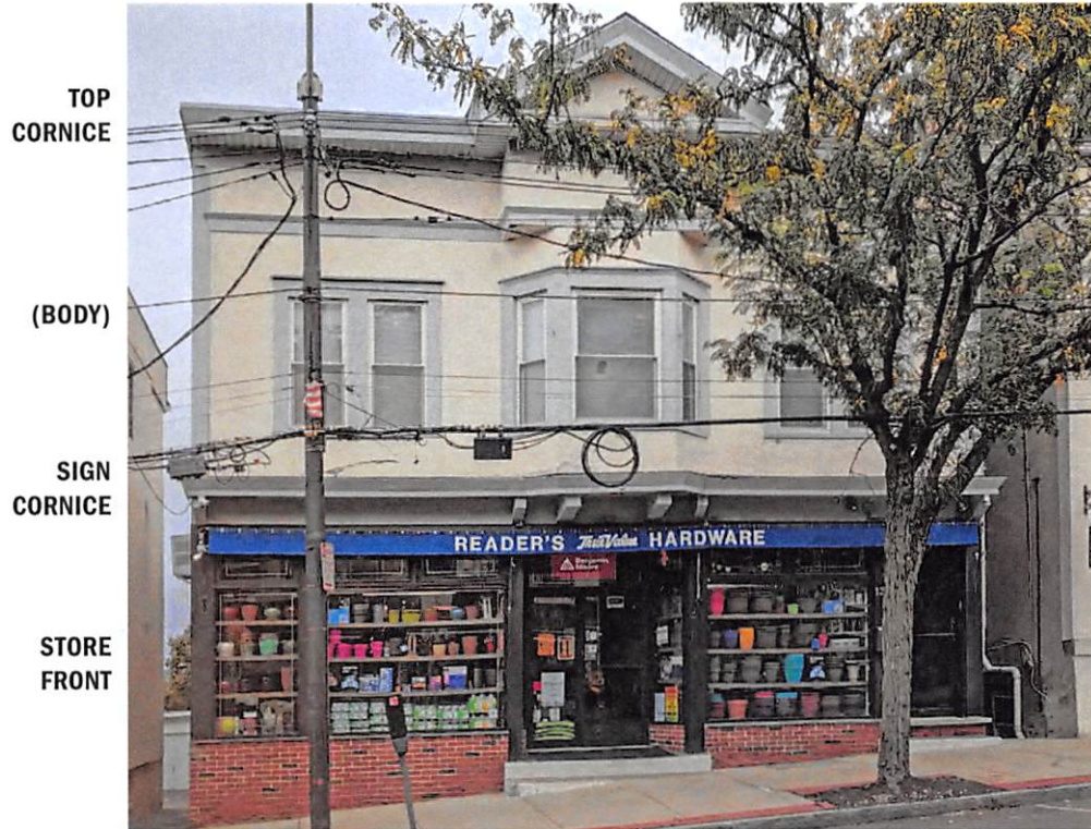
The classic American downtown building arrangement includes an upper cornice, windows for the “apartments over the store” a sign cornice and more horizontal detailing over a glassy, ground level retail frontage with a recessed entry.
