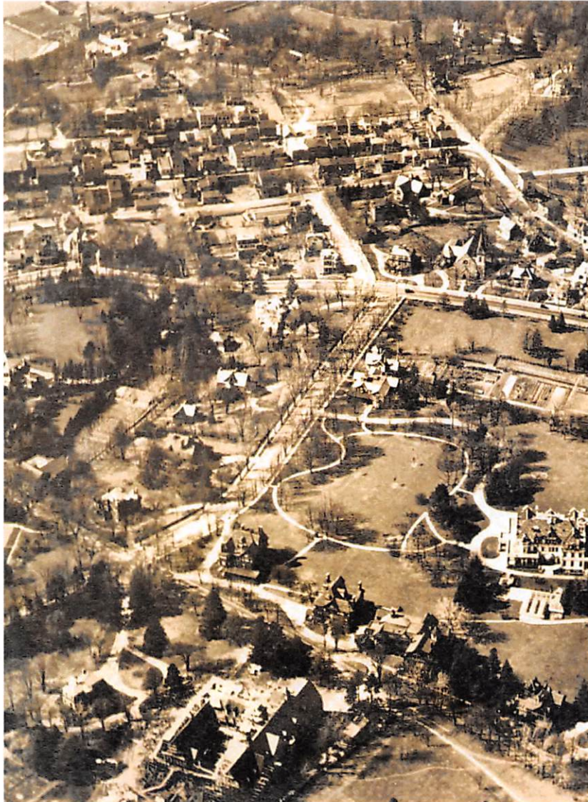
1920s aerial photograph: Looking from above construction underway at the Masters School down Clinton Avenue to Broadway, Oak and Elm Streets, the Old Croton Aqueduct, Main Street, Cedar Street, Palisade Street, and at the top of the picture, on the Hudson, the brewery that gave way to the Methodist Book Concern (now 145 Palisade Street) in October of 1927.
