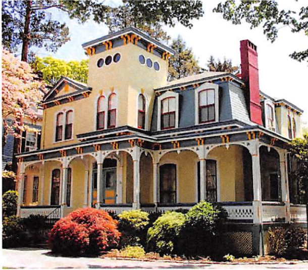
A mansard roof adds a Second Empire touch to an asymmetrical composition with both flat and round arches.
