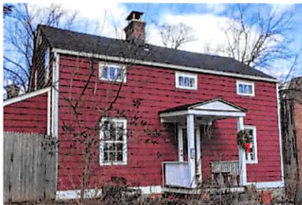
This three bay example with center chimney has faced Broadway (the "Highland Turnpike" in 1859) for over 150 years.
